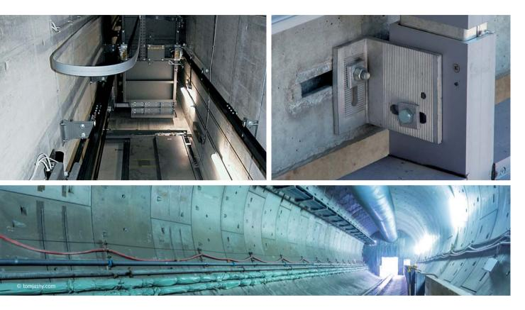
Available from HALFEN as of January 2017, the new anchor channels with extra load capacity. We set new standards in load classification with the HTA-CE 40/22P and HTA-CE 50/30P. Thanks to intelligent engineering the new channel profiles provide up to 45% more capacity through optimized use of material.
